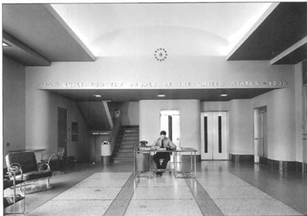
Reception Room Pickwick Dam 1939
